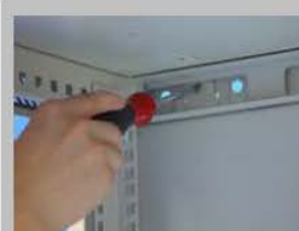
Inside fixation by nuts to avoid accident
