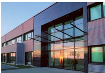
MEISINGER Headquarters Neuss, Germany
