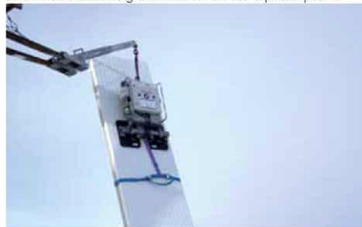
Picture 20. Lifting a correctly secured panel with vacuum cups and belts.
