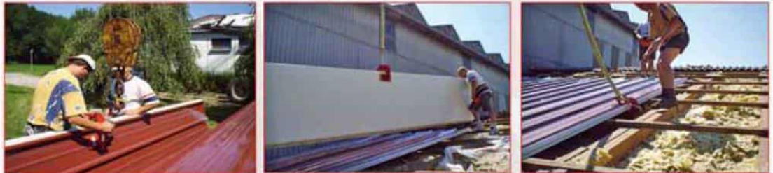
Picture 26. Stages of transportation of roof panels with the help of a self-locking assembly tool.
