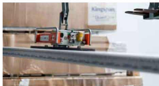
Picture 19. Positioning the elevator on the top/first panel.
