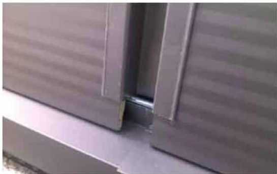
Picture 69. Drainage channel for K175 Top-hat dressing (bottom) and sample installation point (top)
